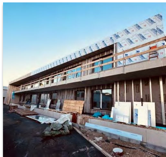
Construction site new building
